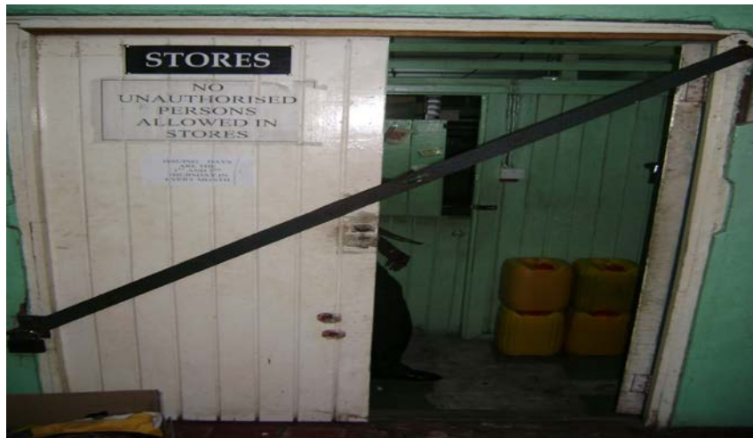
Fig. 5 – MLHSSS Entrance to Stores (Photographed 29/09/09)
